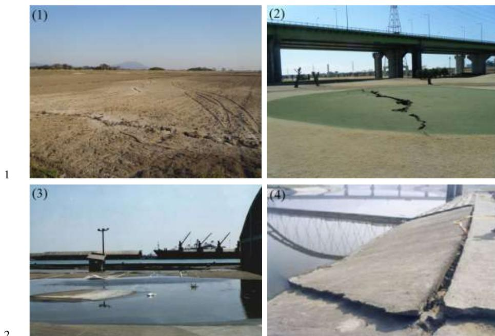
4 Figure 5. Photos showing liquefaction-induced hazards during the Chi-chi earthquake
