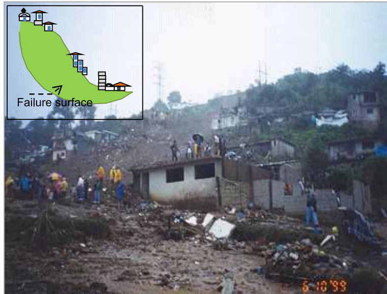
Figure 10. Elements at risk within the failure block (La Aurora landslide, Teziutlán Puebla, México).
